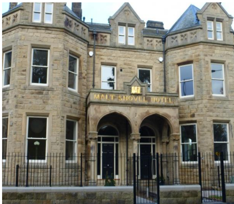
The Malt Shovel an example of a former hotel within Burley adapted for new residential use.
